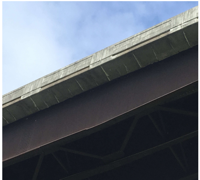
PHOTO 2 Description Typical cracking in the overhangs.
