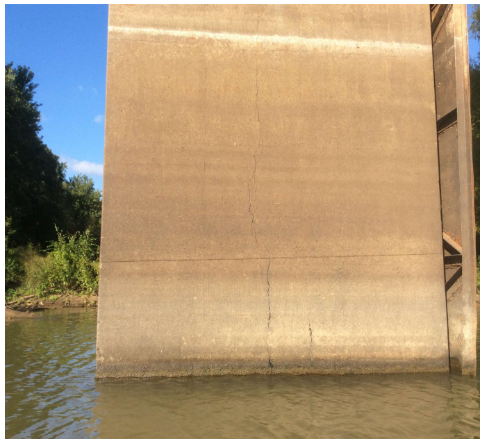
PHOTO 1 Description Pier 13 vertical crack on ahead side up to 1/4" wide extending up about 15' from water line
