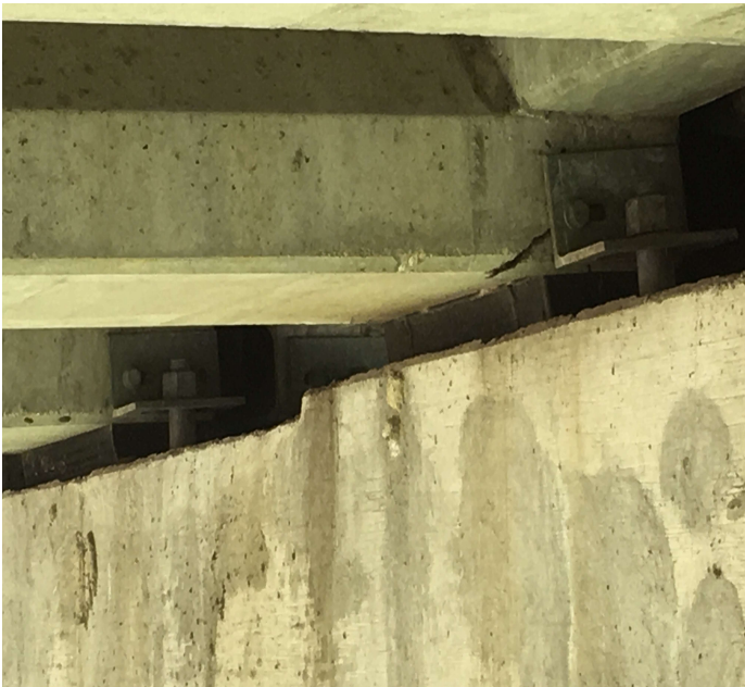
PHOTO 4 Description Bent 7, Girder 3: Spalling in the bearing area.
