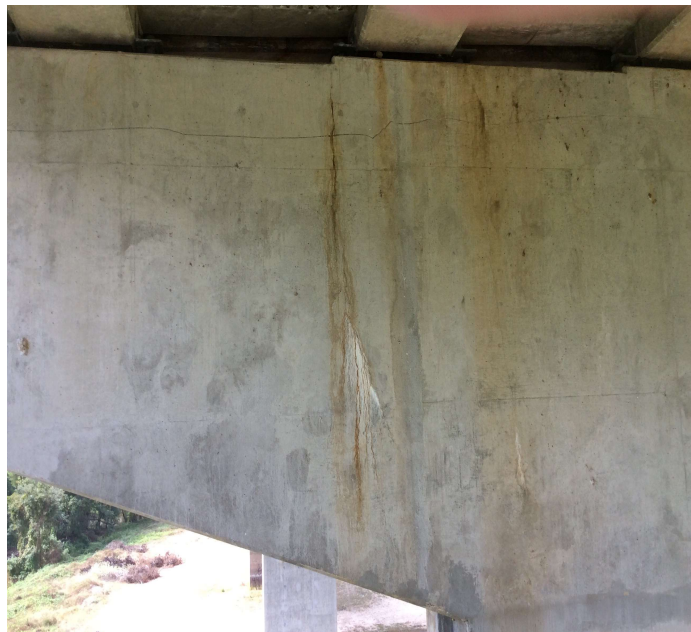
PHOTO 1 Description Bent 7 vertical hairline shrinkage crack in face of cap typical with all bent caps.
