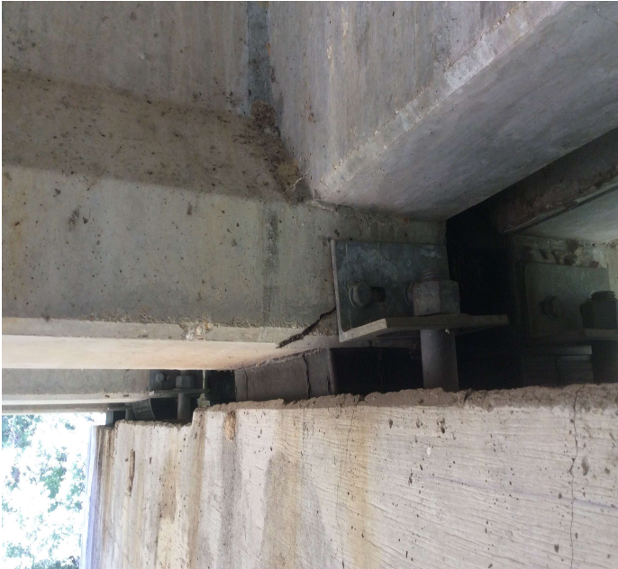
PHOTO 3 Description Bent 7 girder 3 crack in bottom flange where anchorage system is attached.
