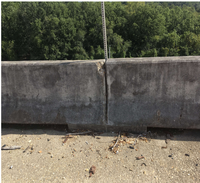
PHOTO 1 Description Span 24, Right, Bridge Rail: Spalling.
