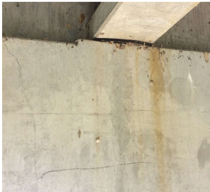
PHOTO 1 Description Bent 6 girder 4,5,6 bearing pad is working out of place.
