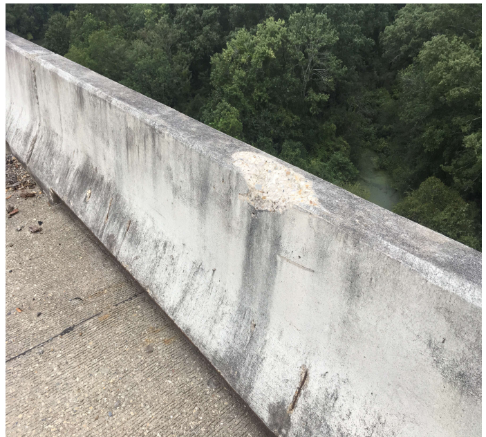
PHOTO 2 Description Span 16, Left, Bridge Rail: Spalling.
