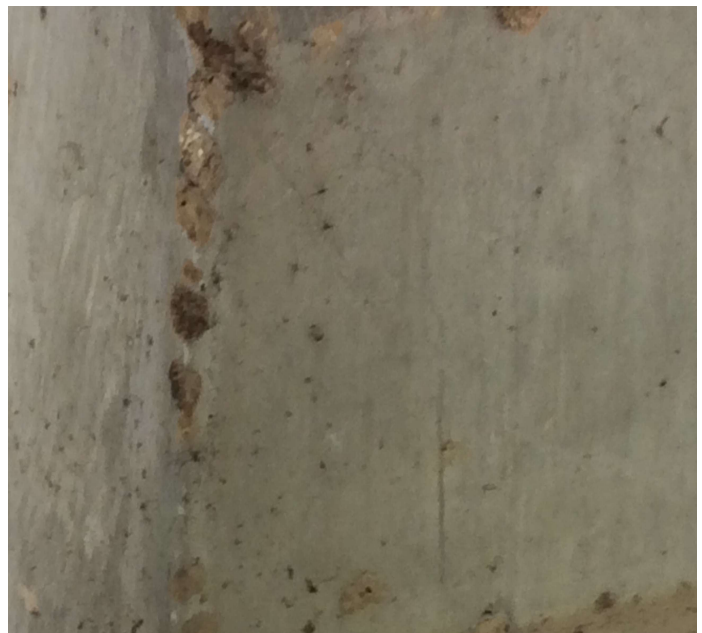
PHOTO 2 Description Bent 11 girder 4 diagonal crack in web of girder in bearing area.
