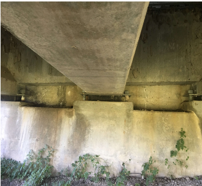
PHOTO 1 Description Bent 26: Isolated diagonal and vertical cracking with light efflorescence.
