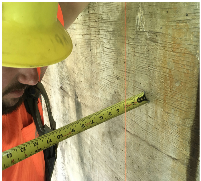
PHOTO 2 Description Bent 20: Offset cap.
