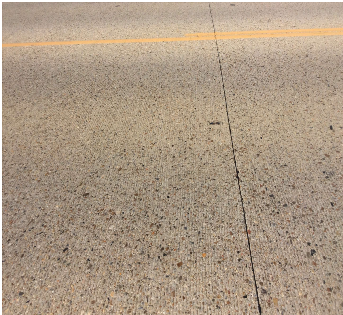
PHOTO 1 Description Sealable deck cracking at random spacing. Typical
