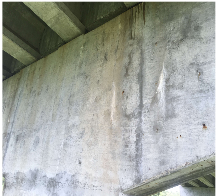
PHOTO 2 Description Bent 20, Cap: Cracking with efflorescence.
